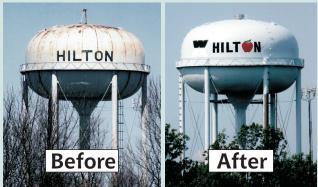
After 4,500 man hours of labor over the course of 4 months, using over 900 gallons of paint inside and out, the water tower project is finally complete!
